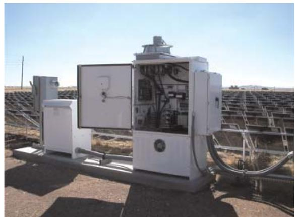
Figure 3. Xantrex PV150 system inverter
